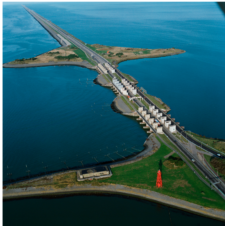
Figure 1. Coastal infrastructure is intended to function for multiple decades. Level control facility in the Netherlands, constructed in 1932 (Image: Rijkswaterstaat image library).
